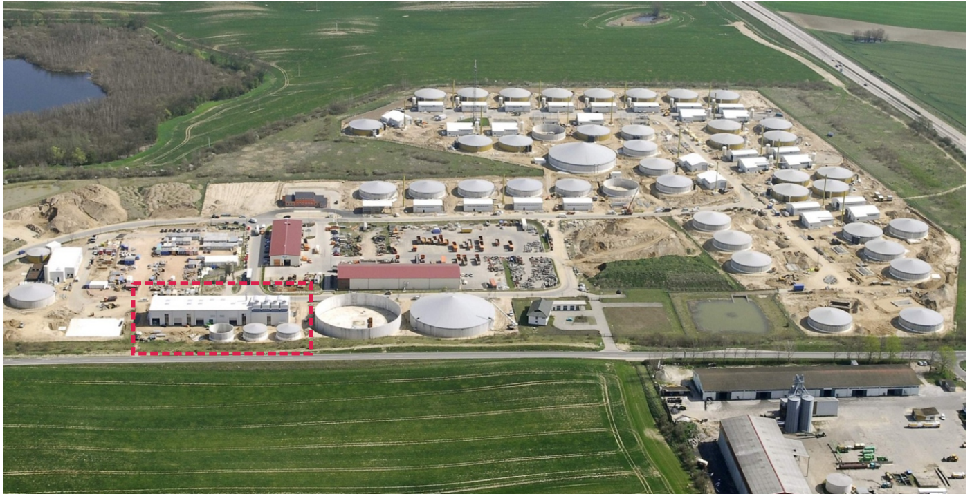
GÄRREV plant for bioenergy park "Klarsee", Germany, approx. 20 MW el /h
